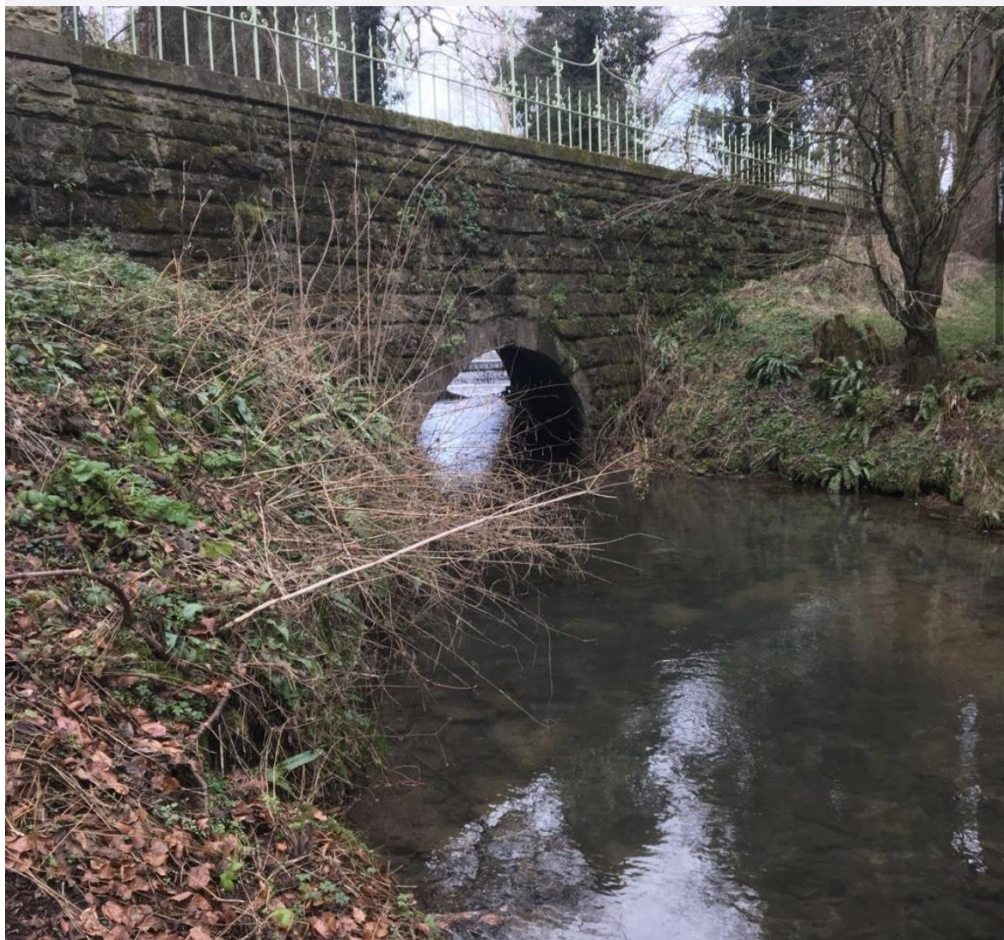
Fig 1.5 Photos of Cowley Bridge
