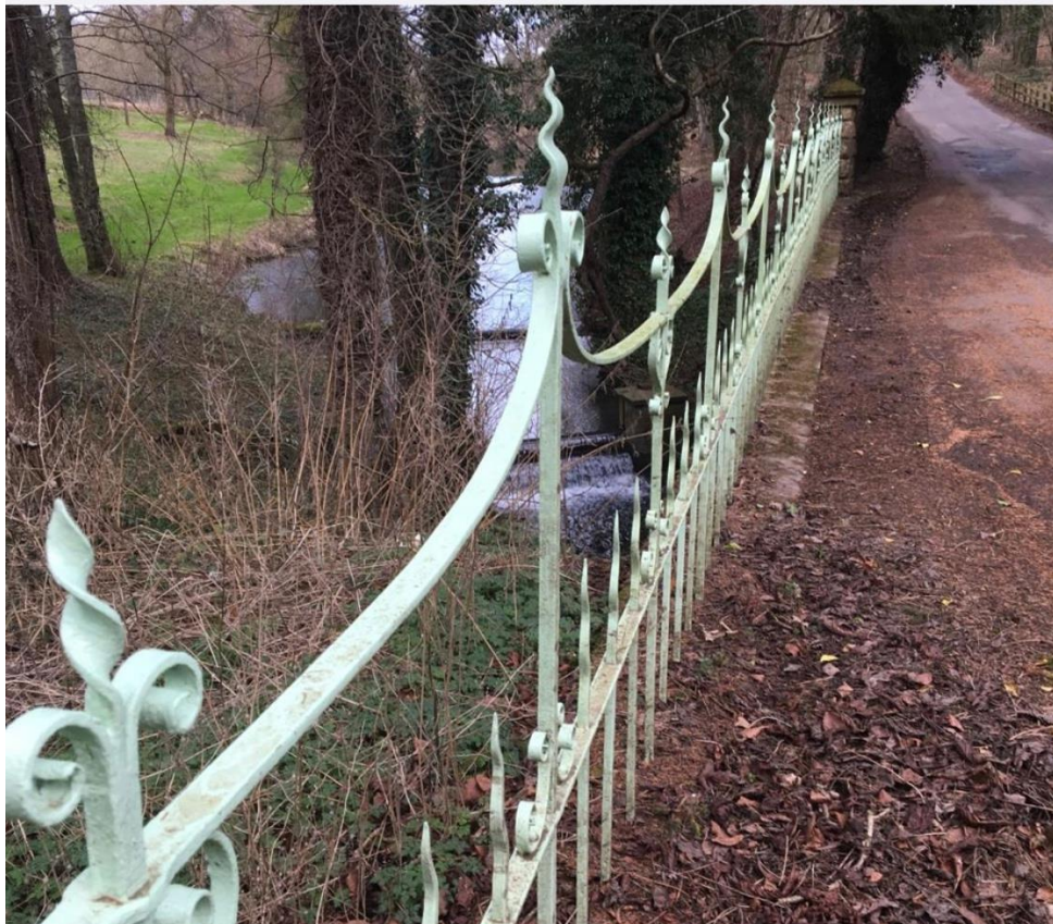
Fig 1.6 Photos of Cowley Bridge
